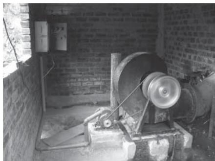
Figure 3 The low-head turbine at Magdalena drives an induction motor as generator (IMAG) with controller (photo: Robert Simpson)
