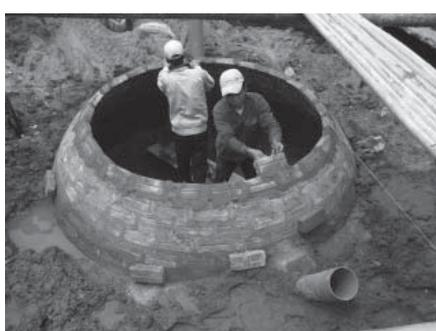
Figure 2 Construction of a biogas plant (photo: Biogas Programme Vietnam)
