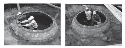
Figure 2 Construction of a biogas plant (photo: Biogas Programme Vietnam)
