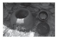
Figure 9 The opening for firewood is marked in the moist earth. The opening will be removed after a day. (*photo: Peeyush Sekhsaria*)
