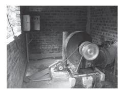
Figure 3 The low-head turbine at Magdalena drives an induction motor as generator (IMAG) with controller (*photo: Robert Simpson*)
